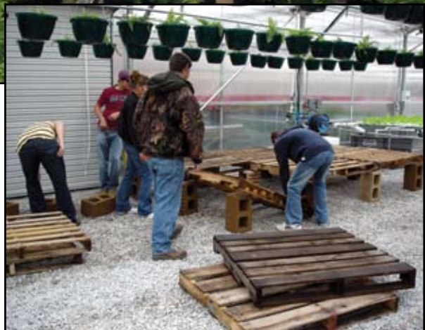
Students use discarded wooden pallets and concrete blocks to build inexpensive platforms for growing and selling poinsettias.
