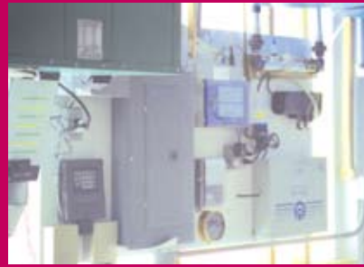
CropKing supervised installation of controls and pumps used to operate the NFT system at the Manatee greenhouses.
