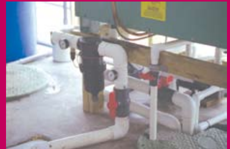
CropKing supervised installation of controls and pumps used to operate the NFT system at the Manatee greenhouses.
