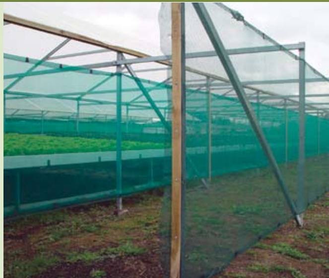
Above left: Raw water is pumped from an underground bore and enters the iron/manganese treatment cylinder shown at right. The hardness is adjusted by pump injecting a softener (center) and then enters the reverse osmosis unit (left). Above right: Most of the 25 growing structures on the site follow this simple design. High-tensile rectangular hollow section framework is roofed with horticultural plastic film. The sides are covered with standard shade/wind break cloth. This particular house is exposed to the open ground.
