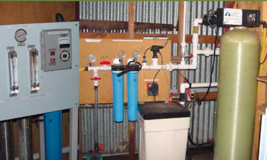
Above left: Raw water is pumped from an underground bore and enters the iron/manganese treatment cylinder shown at right. The hardness is adjusted by pump injecting a softener (center) and then enters the reverse osmosis unit (left). Above right: Most of the 25 growing structures on the site follow this simple design. High-tensile rectangular hollow section framework is roofed with horticultural plastic film. The sides are covered with standard shade/wind break cloth. This particular house is exposed to the open ground.
