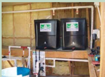
Left, top to bottom: The signage above the drying tunnel entrance says it all for me. Sun Valley Produce staff are constantly reminded of the high standards expected by clients. A Sta-Rite centrifugal hydro pump, my favorite, supplies nutrient out to the beds. A and B nutrient concentrate containers, filters and solenoid valves dump concentrate into the main tank to maintain the desired CF value. Above: The washed product continues along a motorized conveyor through this refrigerated, fan-assisted drying tunnel to the packing benches. It then goes into cool stores awaiting transport to clients. Nothing stays around for very long, and temperatures are never allowed to rise.
