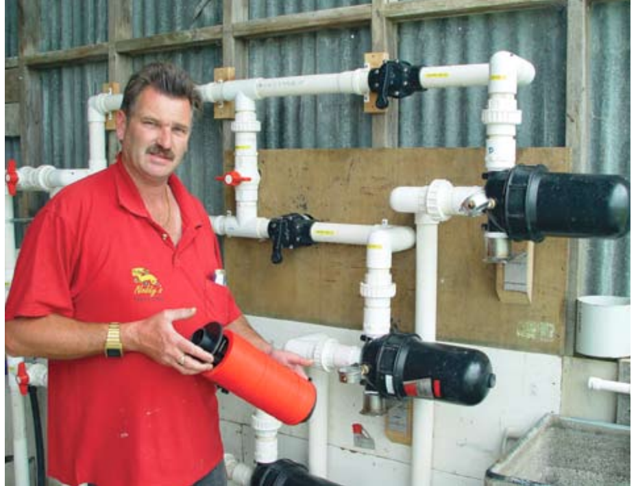
Above: Noddy keeps a cleaned cartridge ready to aid rapid replacement to avoid any shut down delay to the system when a filter needs cleaning. Below left: Diesel-powered standby alternator. Noddy produces beautiful natural strawberry ice cream with this ice cream machine.
